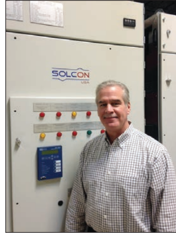
Power play. Solcon USA President Tom Jaros, standing by part of the equipment his company built to control a 12,000 volt motor used by a liquefied natural gas producer in Russia. Solcon recently tripled its floor space by relocating to Cranberry Business Park.
