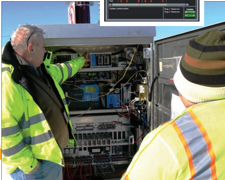
Thinking outside the box. Cranberry traffic signal electrician Marty McKinney shows a Purdue researcher the inner workings of a Township signal control box where a rich trove of data, collected from nearby sensors, is stored.
